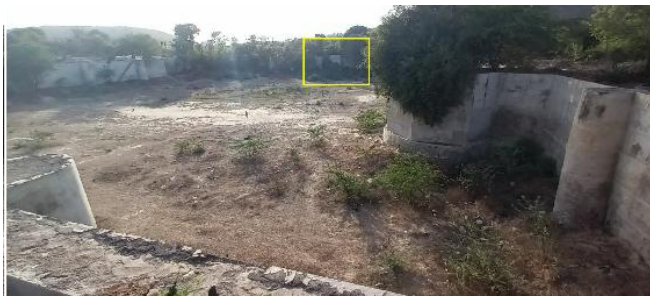
Figure 15. Dohani Kund in a dried-up state with the entrance culvert blocked with vegetation, April 2023. (Source: Author)
