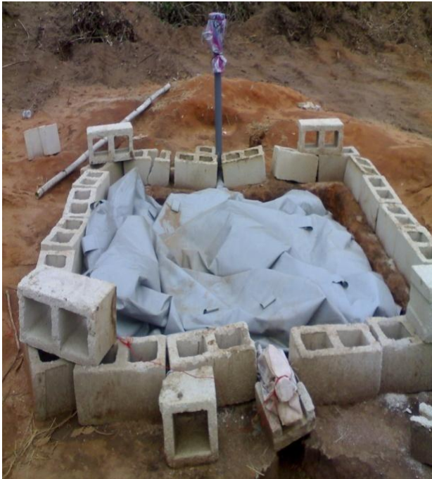
Plate 1: Floating type biogas digester
